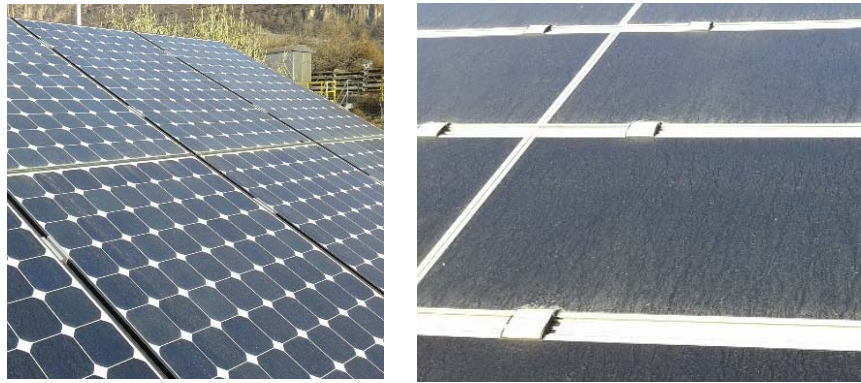
Figure 1: Two of the twenty-four technologies considered in this abstract, visibly affected by soiling.
