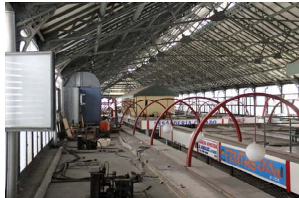
Figure 2: Mercado del Val (Valladolid), interior building view. Source: www.commonenergyproject.eu
