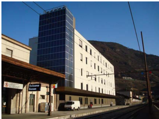
Figure 2: Façade-integrated PV, Ex-Poste building
