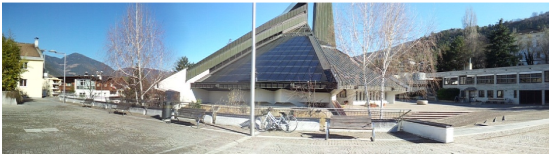
Fig.1. PV roof installation at Milland Church in Bressanone, Italy
