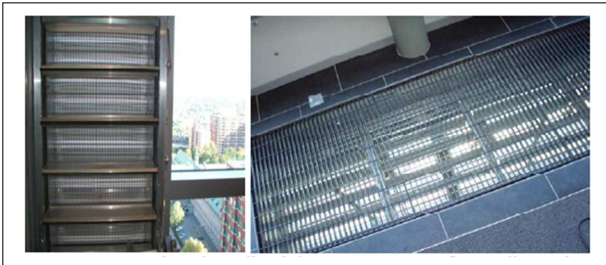
An example of corridor inlet vents (left) and atria connecting floor vents (right), installed for natural ventilation of the Concordia University building in Montreal (Canada)
