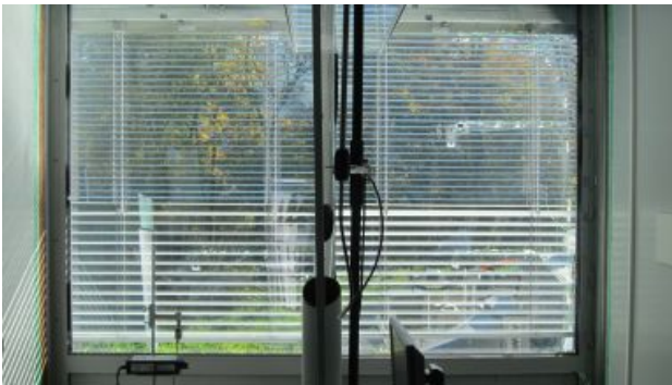
Figure 5: Installed monitoring facade at PASSYS-cell
