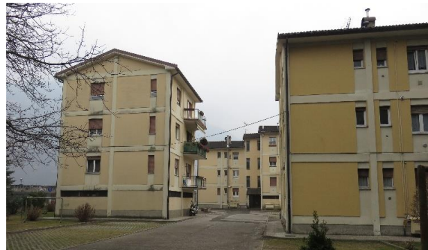
Figure 4. Third reference building.
