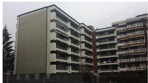
Figure 2. First reference building.
