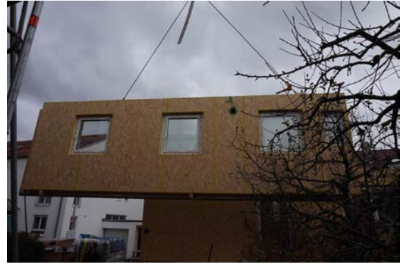
Fig. 4 iNSPIRE façade installation sample, internal side view (source: Gump & Maier)
