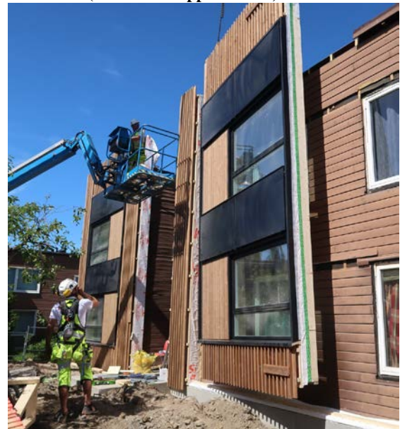
Fig. 4 iNSPIRE façade installation sample, internal side view (source: Gump & Maier)
