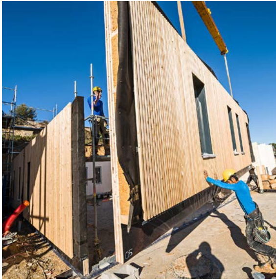
Fig. 11 Façade installation process for the Nexity Ywood «L’Ensoleillée II» building in Aix-en-Provence (source: ©Nexity, Yann Bouvier)
