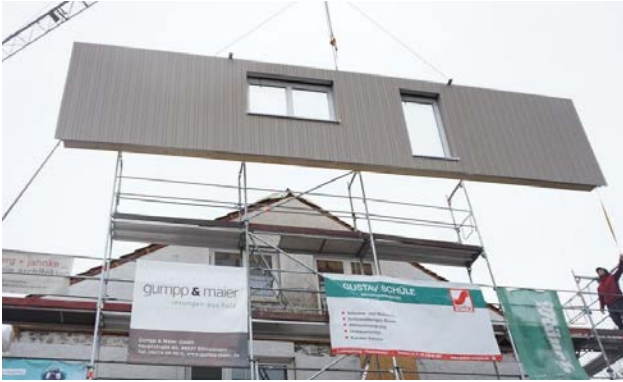
Fig. 3 iNSPIRE façade installation sample, external side view (source: Gump&Maier)
