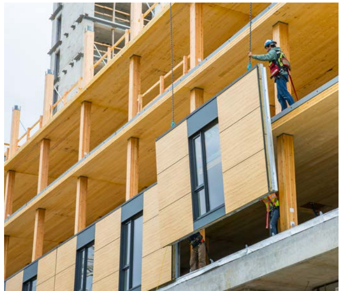
Fig. 12 Brock Commons fully prefabricated envelope installation phase (source: www.naturallywood.com)
