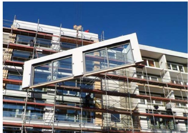
Fig. 2 TES EnergyFacade project – panel installation (source: Gump & Maier)
