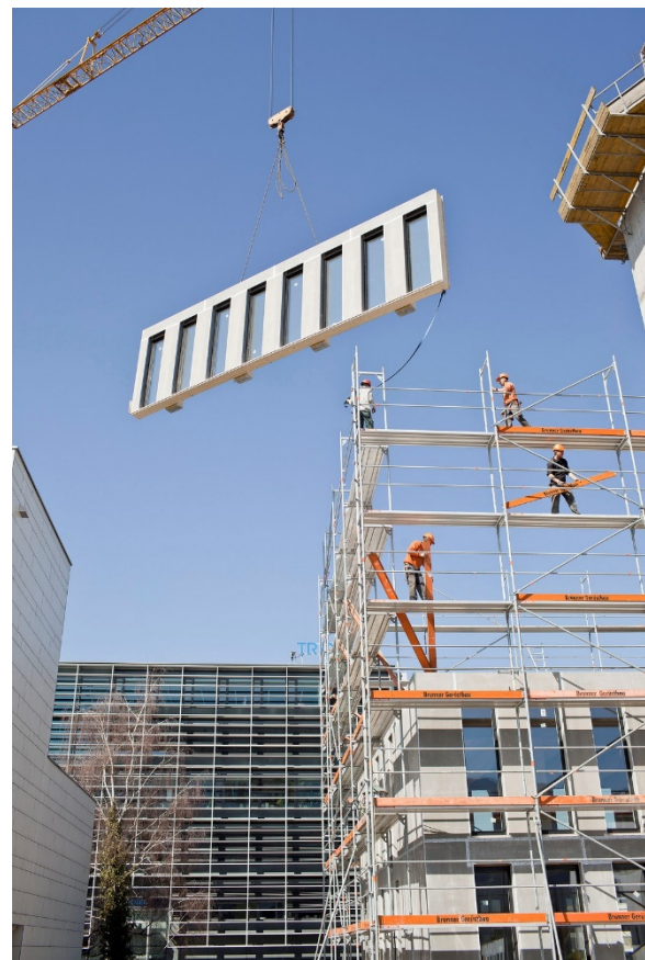
Fig. 10 Installation of LCT ONE façade system through scaffolds (source: www.creebyrhomburg.com ©Darko-Todorovic|Photography|adrok.net)
